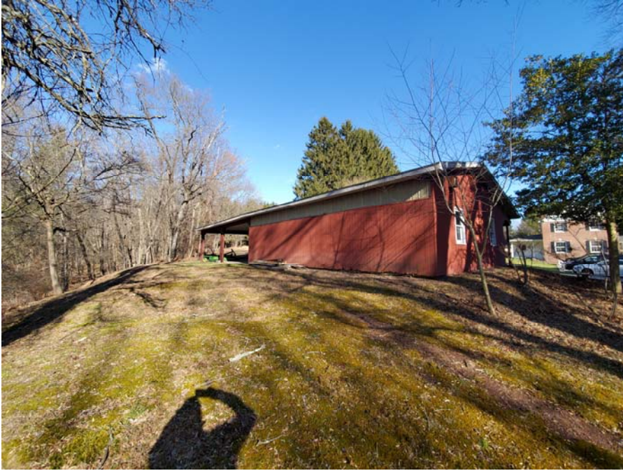
Exterior View of Rear Wall
