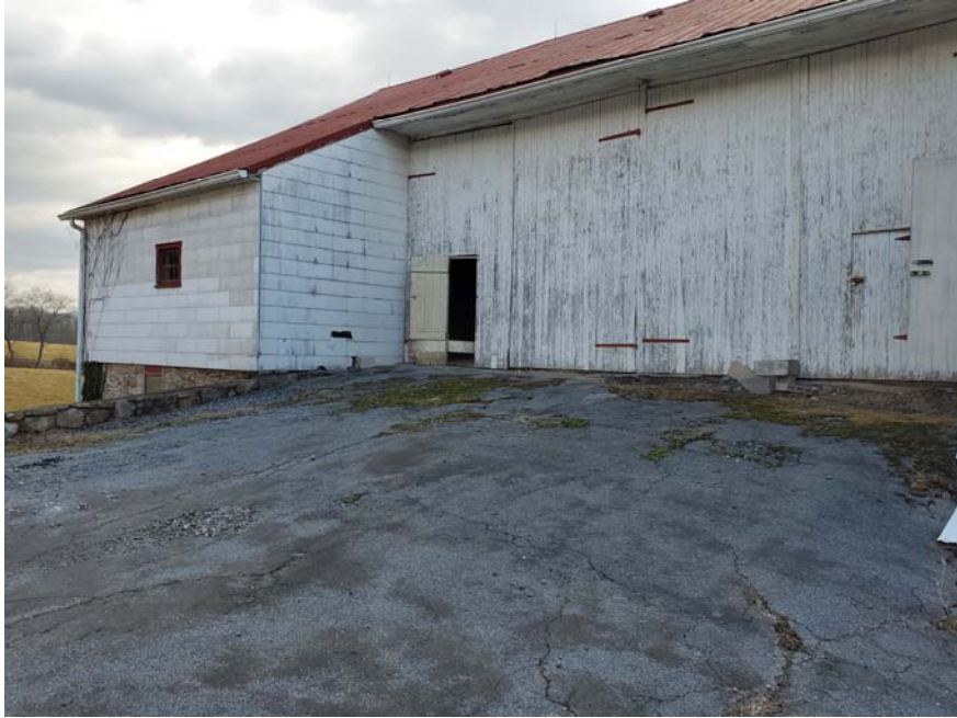
Entrance Doors at top of Bank Ramp
