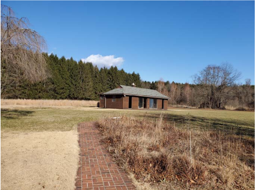
Exterior from South-West (with Brick Path from House in Foreground)
