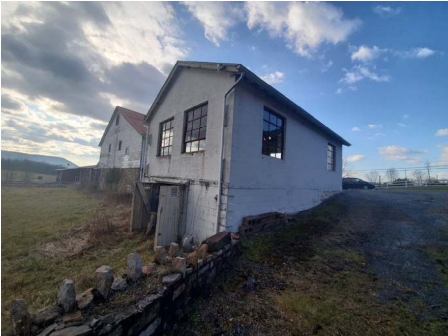
Exterior from North-West
