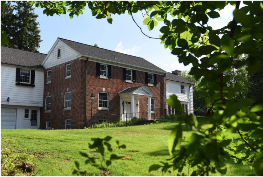
Exterior from South-West (Showing former 1970s addition prior to demolition)
