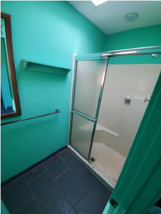
Shower Room Detail
