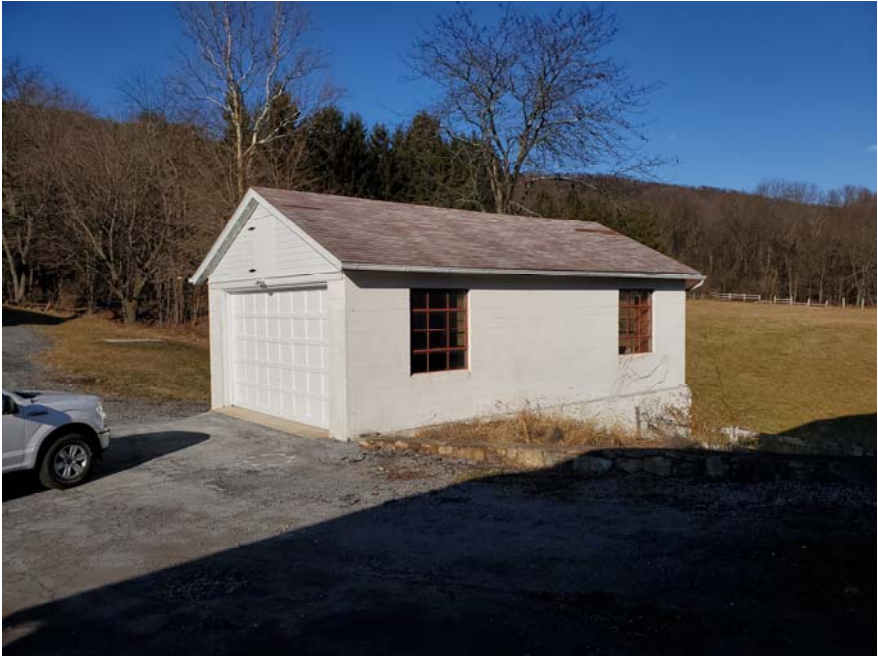
Exterior From South-East
