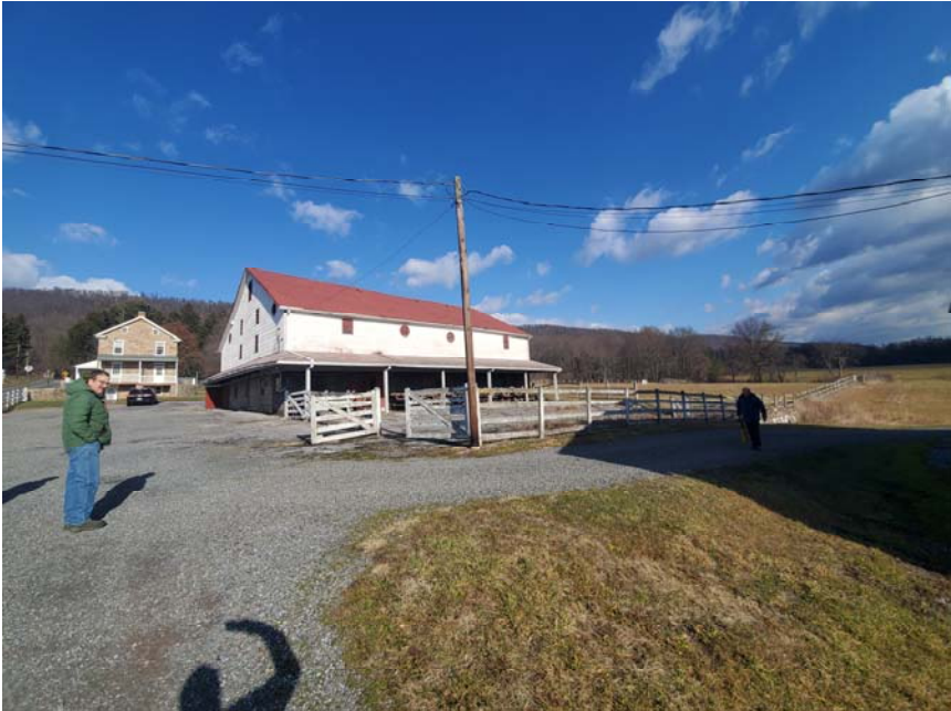
Exterior from South-East
