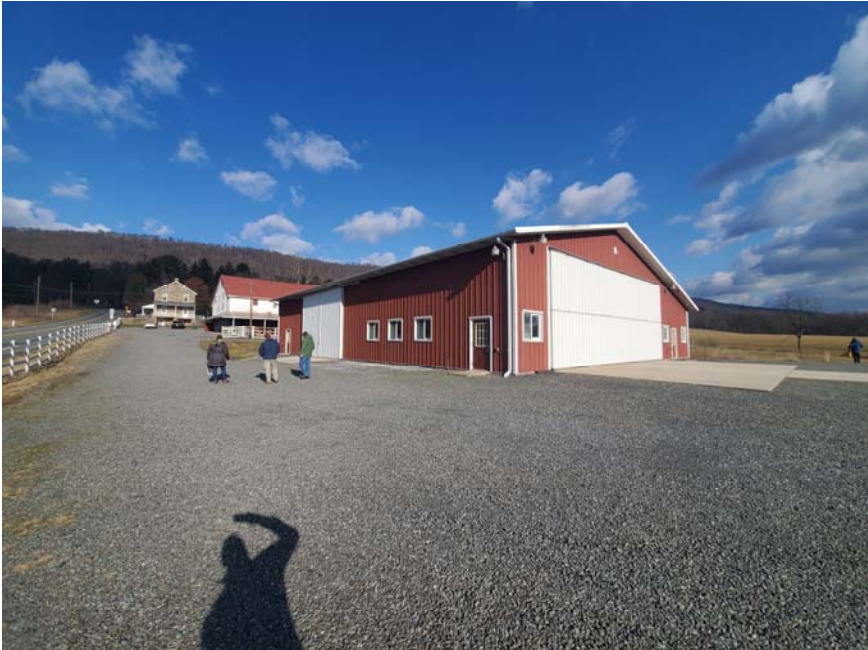
Exterior from South-East
