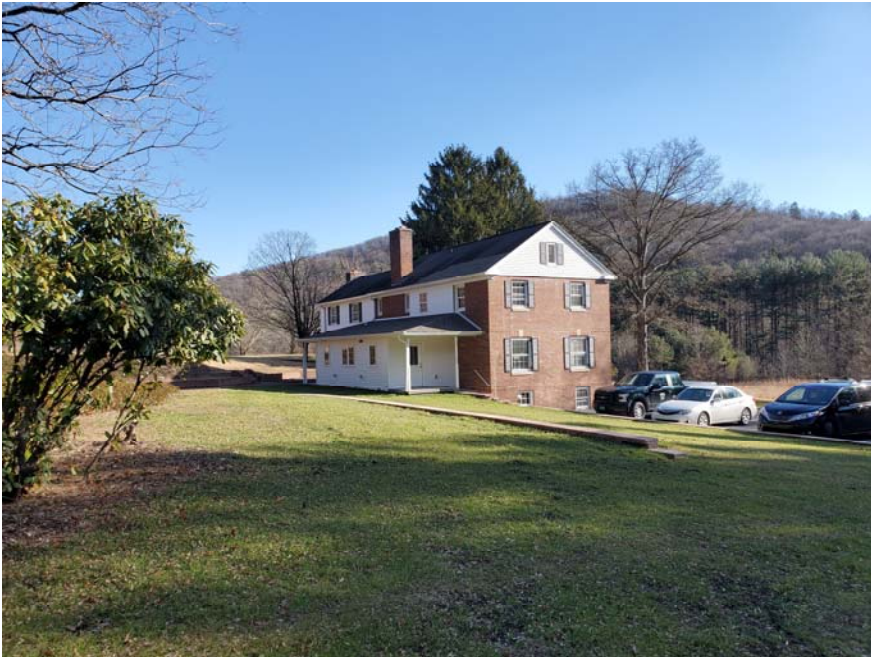
Exterior from North-West (Current State)
