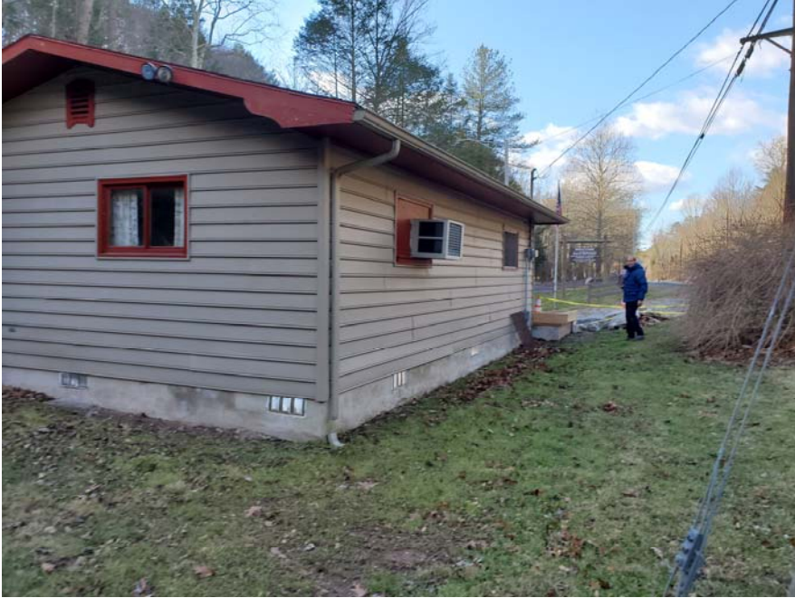
Exterior Corner Opposite, from Entrance, along State Route 325
