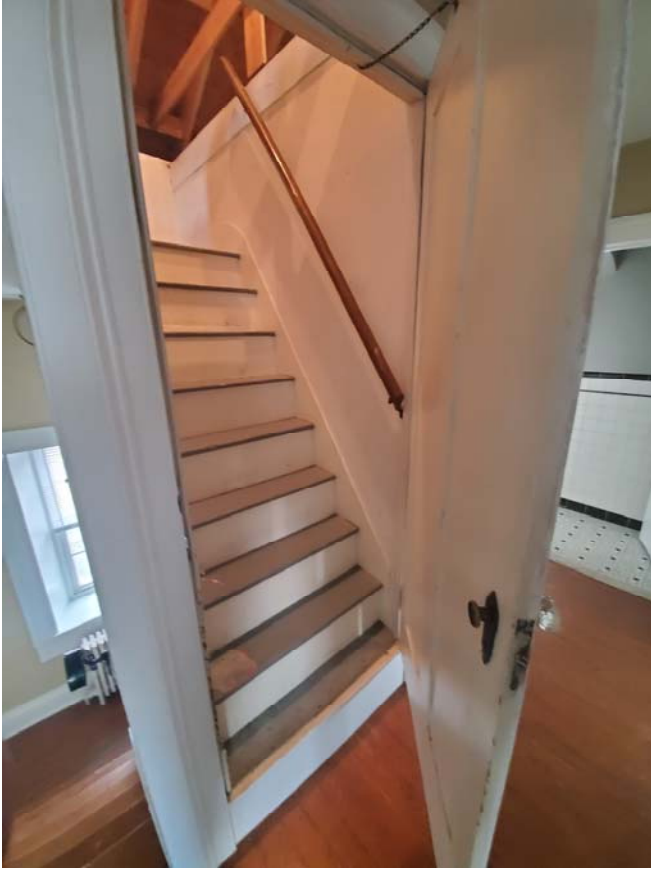
Stairs to Attic
