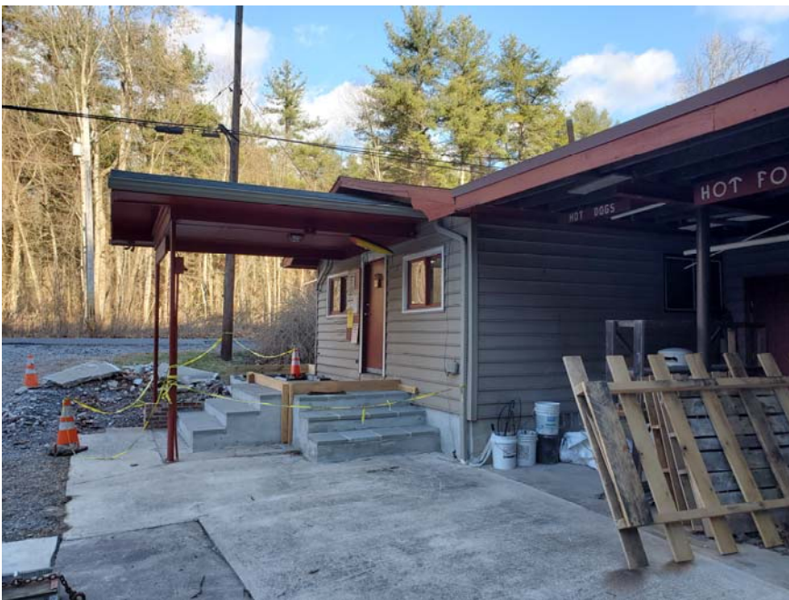
Exterior of new ADA Ramps and Steps at Main Entrance
