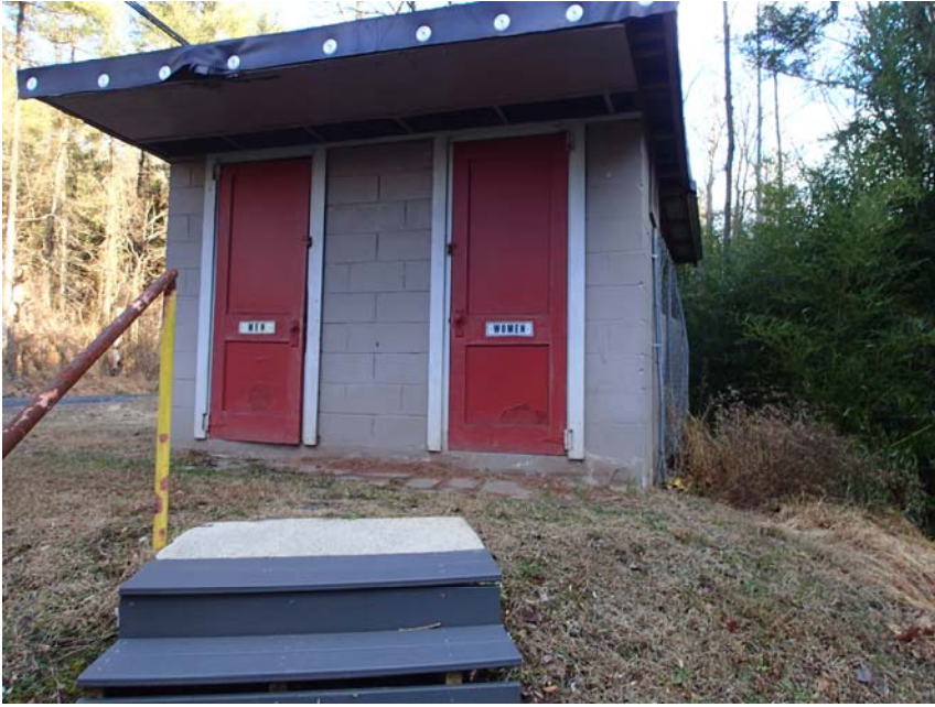
Outdoor Toilet Rooms - No Longer in Use
