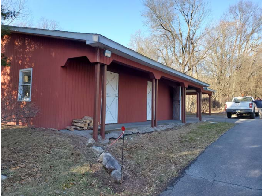
Exterior View of Stable Doors from Driveway
