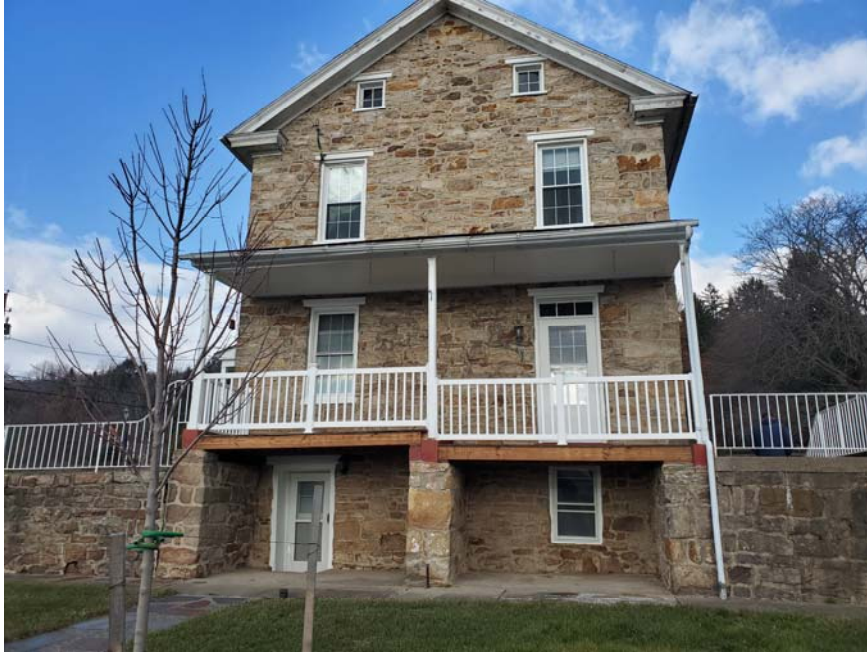
South Façade Showing Porches and Door to Basement Level
