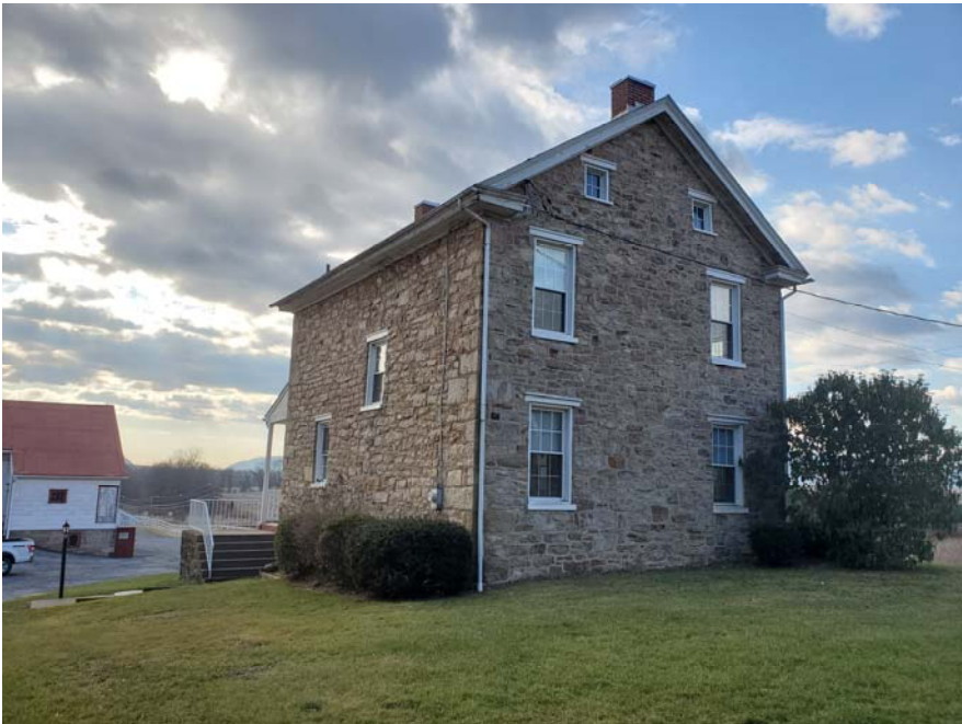
Rear and North Facades
