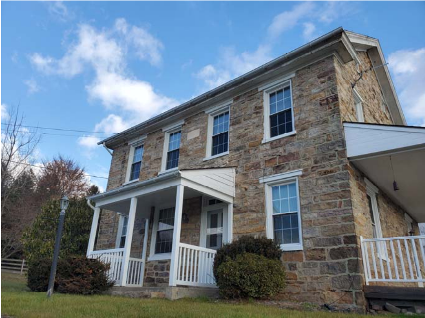
Front Façade from Peter’s Mountain Road
